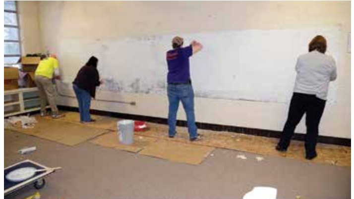
Glenn Hellenga, Jeanne Otey, Mark Vickery, and Cyndy Watts put block fill on a cinder block wall at the Dream Center.
